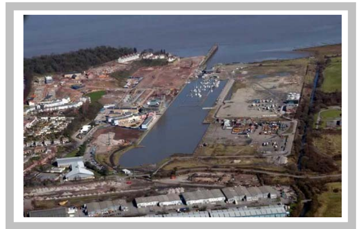
Aerial view of the site under construction
