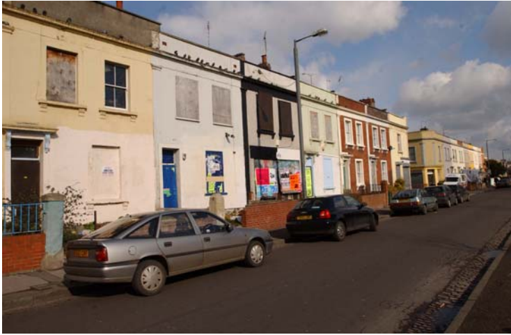
Black and White Café prior to demolition
