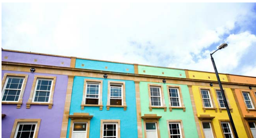
Grosvenor Road, St Paul's – completed scheme
